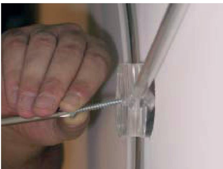
**3.** Fix SpiderX to the wall using the holes in the center of the horizontal crosspiece joints
